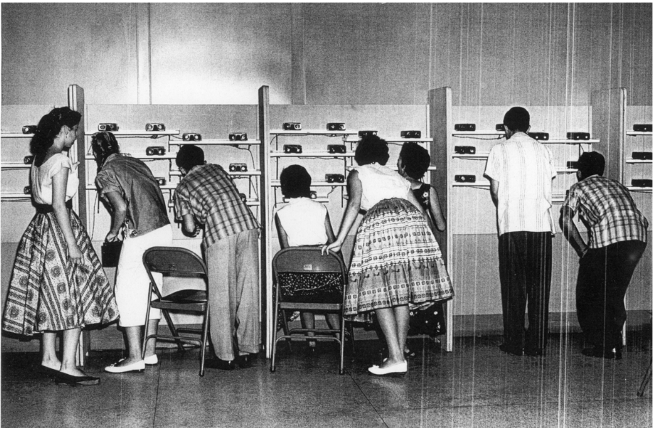
FIG. 3 Built in USA: Post-War Architecture. Installation View. Universidad de Puerto Rico, 1957..
