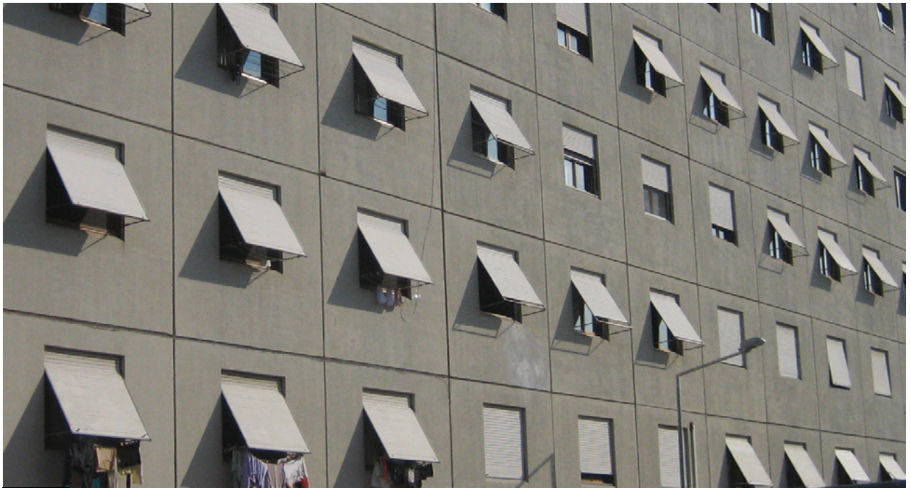
FIG. 26 A building of the district of Valmelaina (N 6), the repetitive sequence of parallel r.c. wall enhanced the semantic of loculus , clearly shown here also in the façade envelope cladding panels
