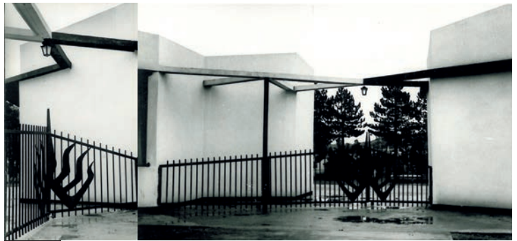
FIG. 12 The principal gate/entrance, meeting the white and black beams, a symbol of the life cycle.
