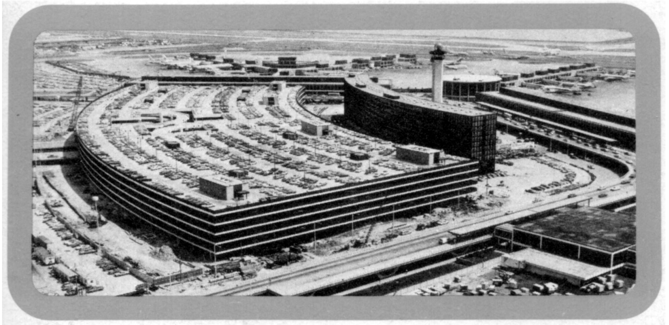
FIG. 9 Parking Garage, O'Hare Airport, Chicago. C. F. Murphy & Associates, 1969. The 'world's largest parking garage,' built to handle the increase in traffic brought about by wide-body jets with over 9000 parking spaces. Contemporary postcard [Author's collection].
