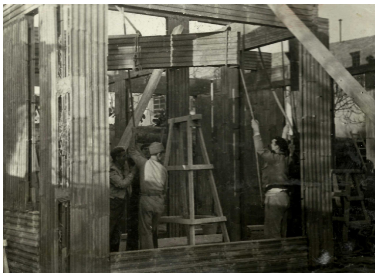
FIG. 10 Javier Modolell LLuch, Construction process: On-site assembly, Madrid, 1948 (Eduardo Torroja's archive).
