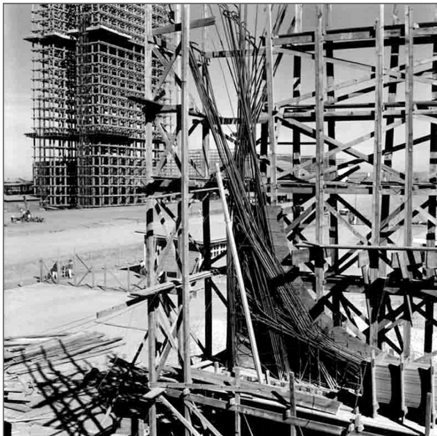
FIG. 11 Palácio do Planalto, Brasília, construction site, 1958. Photo Marcel Gautherot.
