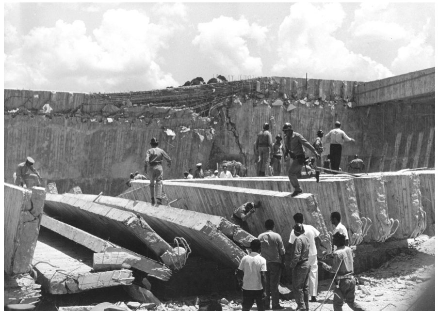
FIG. 8 Gameleira pavilion, Belo-Horizonte, construction collapse February 4, 1971.
