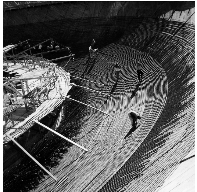
FIG. 12 National Congress, Brasília, construction site, 1958. Photo Marcel Gautherot.
