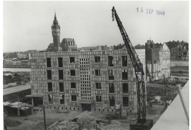
FIG. 14 Société française de Constructions & Travaux publics, Housing block under construction, September 1947 (Eduardo Torroja's archive).
