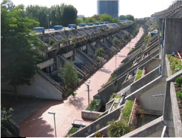
FIG. 7 Alexandra Road, Camden (North London) [Picture taken from: http://www.panoramio.com/photo/16965970 ]
