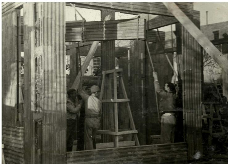
FIG. 10 Javier Modolell LLuch, Construction process: On-site assembly, Madrid, 1948 (Eduardo Torroja's archive).
