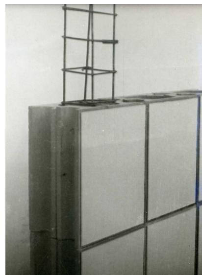
**FIG. 13** Société française de Constructions & Travaux publics, Industrialised concrete blocks. Erection of walls with embedded columns, 1948 (Eduardo Torroja's archive).
