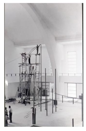
Fig. 8 Installation of metal tubing tracing the line of a ship, designed by Tursini (Nemi Ships Museum archive).
